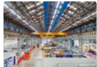
Rolls-Royce – production hall refurb
