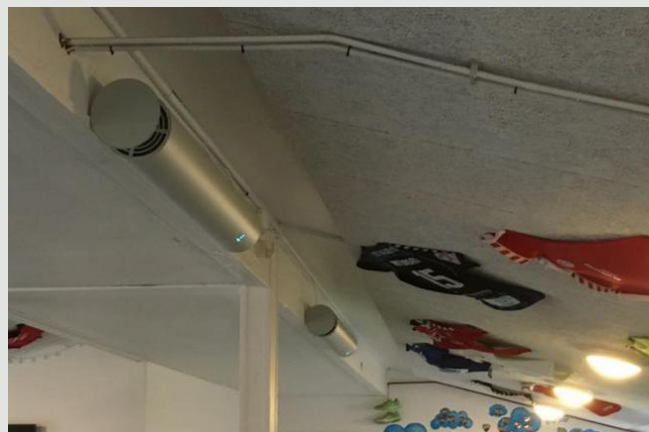
SINE is a sports school in Denmark where students play sports together after school. The school installed Luxibel disinfection systems in the common areas to make sure this could happen in a safer way and lower the risk of coronavirus infection. The B AIRV2s ensure that the air is extensively disinfected and that students can again enjoy sport and relax together in a safer environment.
